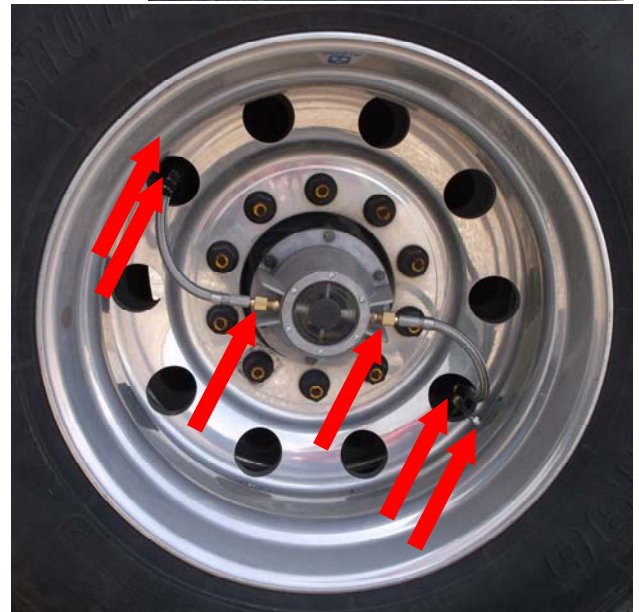
Soap check both ends of each hose, base of each valve stem
